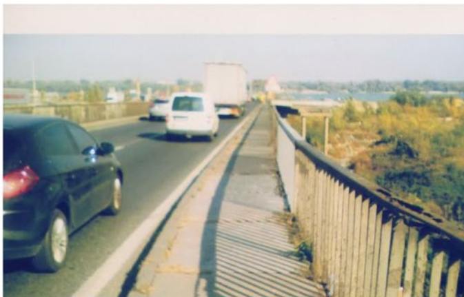
Fig. 1: The appearance of the pedestrian guardrail immediately upstream of the point where the vehicle left the bridge
